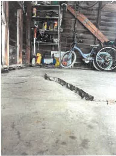
Cracking foundation
