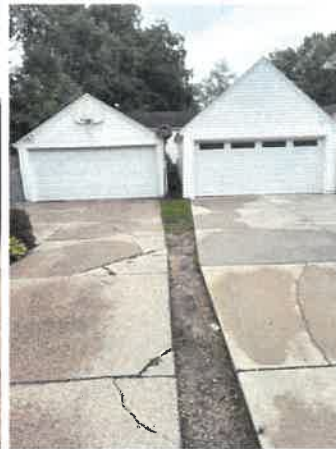
Side by side garages
