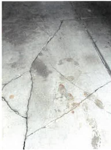
Cracking foundation
