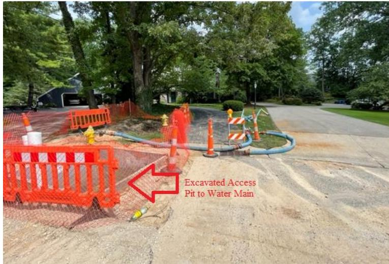
Step 2: The contractor will arrive on site and install an above ground temporary water system which includes above ground main, and service leads to homes. The system is disinfected/chlorinated and tested before residents are switched from the existing water main to the temporary system.
