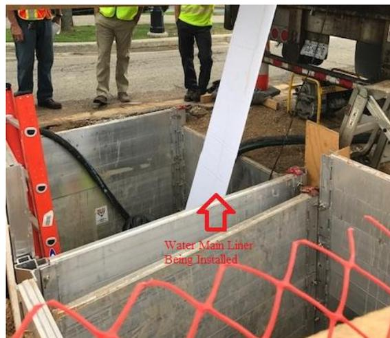
Step 7: EGR Department of Public Works staff will reconnect the rehabilitated water main at access pit locations by installing new valves, tees, crosses, and small segments of water main while the contractor reinstates water services with specialized robotic cutting equipment. Throughout the project EGR Department of Public Works staff will also be replacing any lead water service lines in the project areas in advance of bringing the rehabilitated water main back into service.
