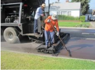
1 Asphalt slurry applied
